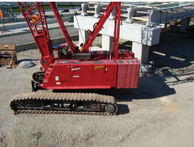
Local contractor - Dan's Excavating
