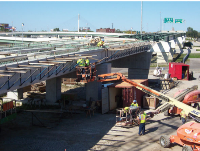
View of on-going work on SO2 ramp
