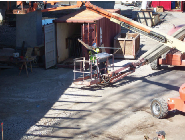
SO2 - View of local contractor working on-site
