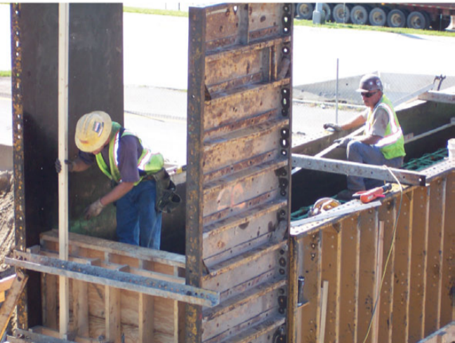
Local contractors working on pier cap form
