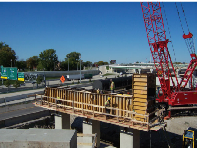
View of pier cap form on top of concrete columns
