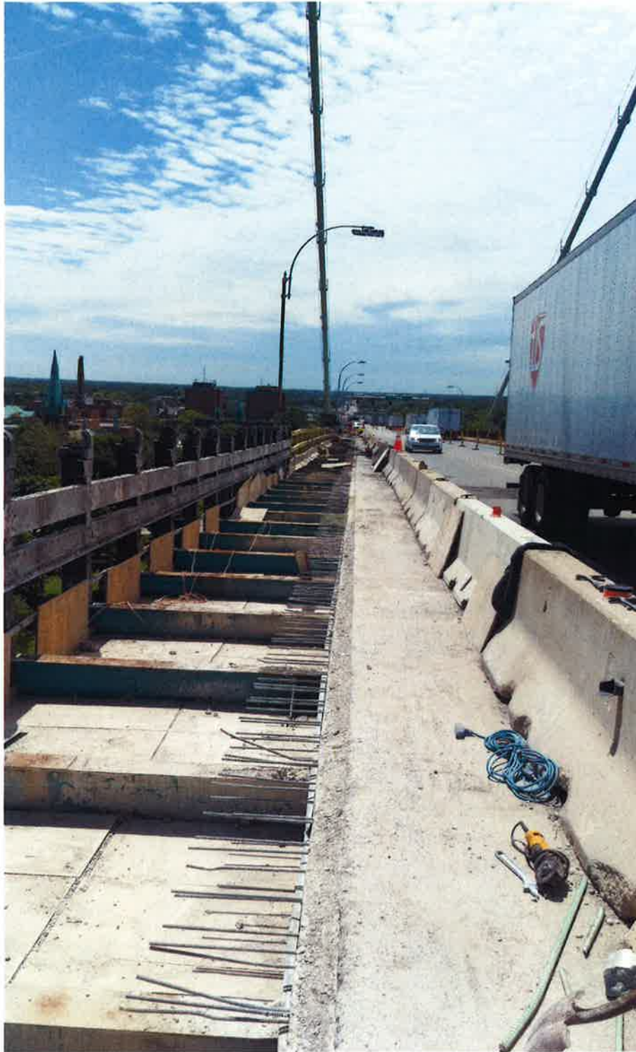
Old railing removed up to CC2 joist 18
