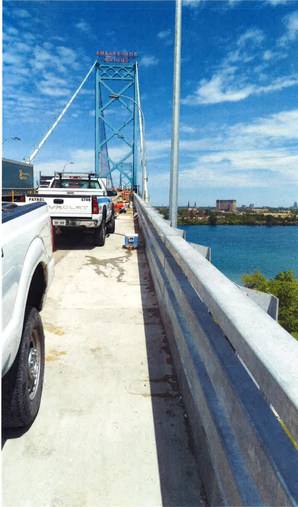
Rail complete up precast panel 14, approximately 304'
