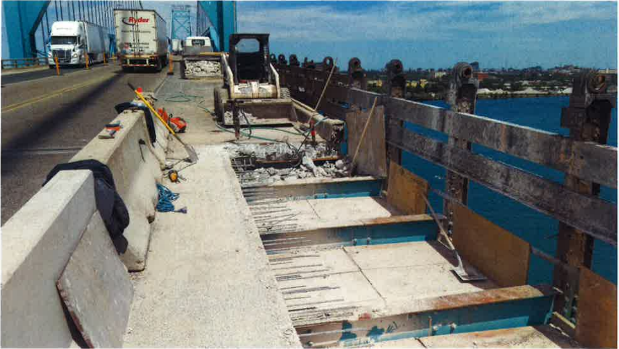
Deck removed up to expansion joint at end of CC2
