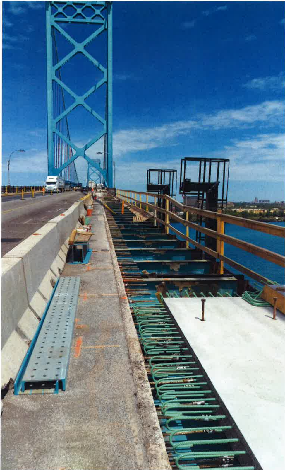
Old railing removed to CC2 joist 18
