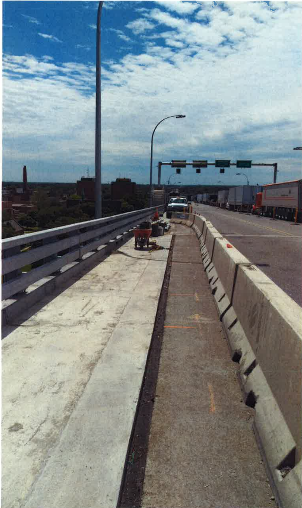
Ready to relocate 100' of barrier up to CC4 joint 7
