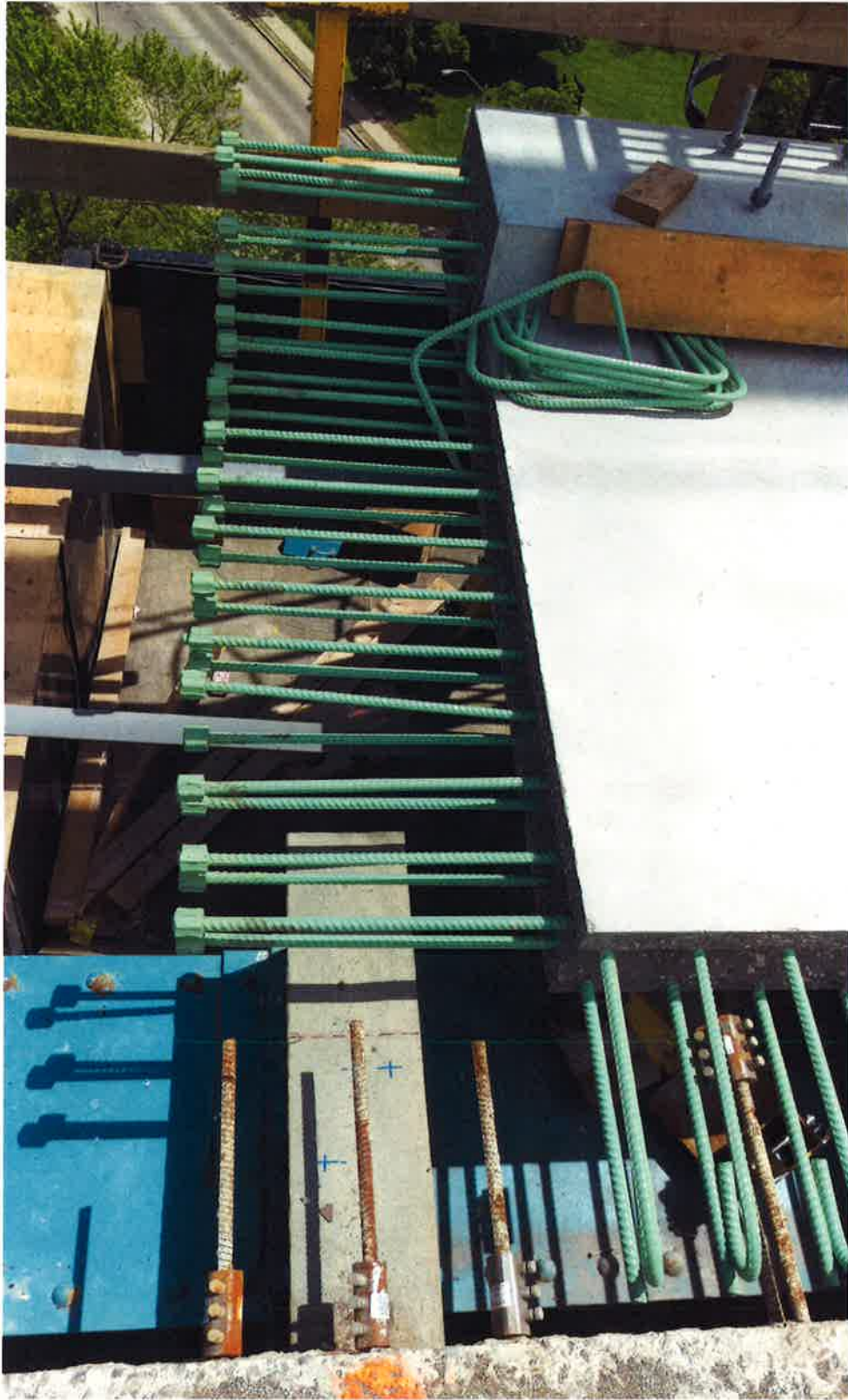
Precast Panel 17 & 18. Scheduled to be grouted June 9, 2016
