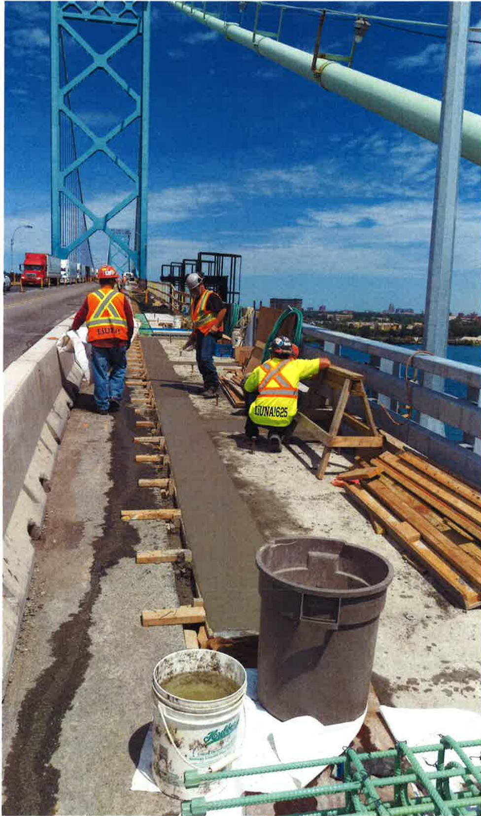
Precast Panel 13 through 16 concrete pour June 9, 2016
